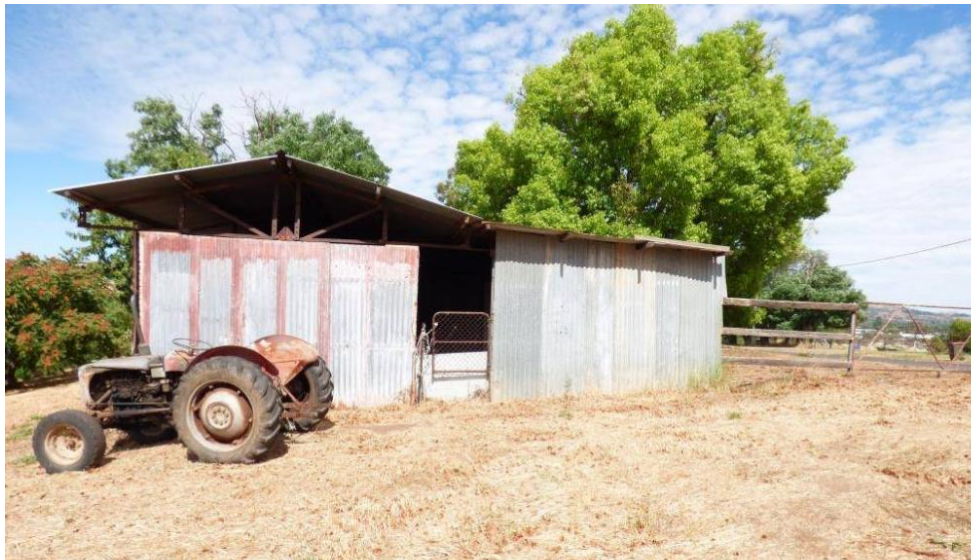
Figure 6 – Shed now demolished, looking from East to West (source:realestate.com)
