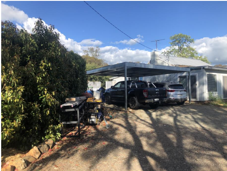
Figure 8 - photo of carport and overhead service line.
