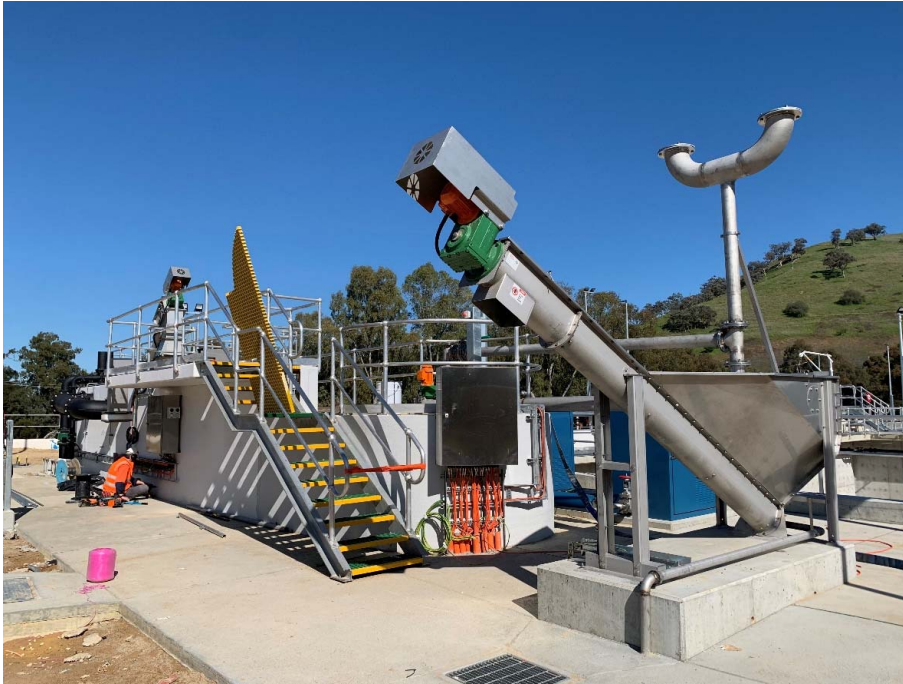
Photo 1: Mechanical installation complete for inlet works.
