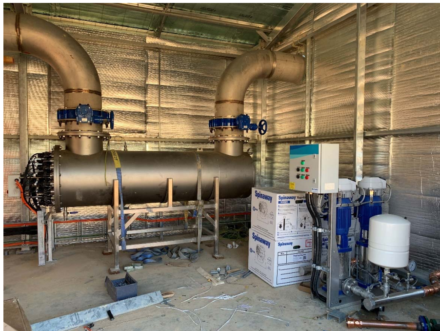
Photo 3: UV disinfection unit installed.
